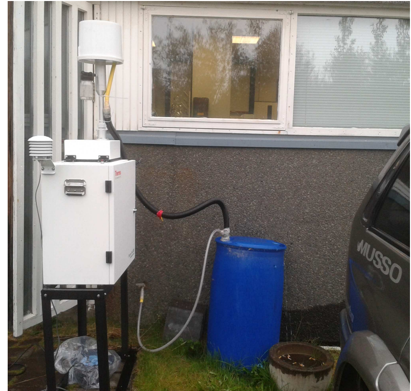
The arrangement for collecting diesel exhaust
